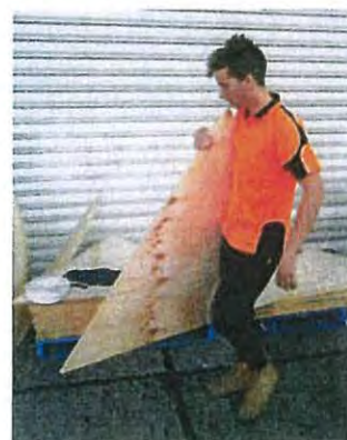
Replacing triangle boards
