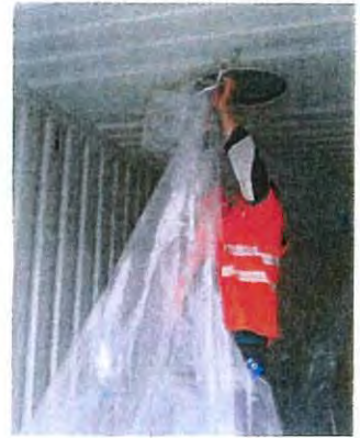
Fixing top liner to central hatch
