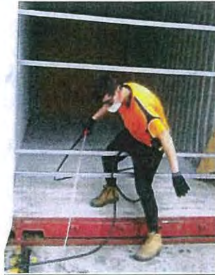
Climbing through entry with compressed air cleaner
