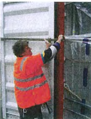
Replacing cross bars and fixing outer liner
