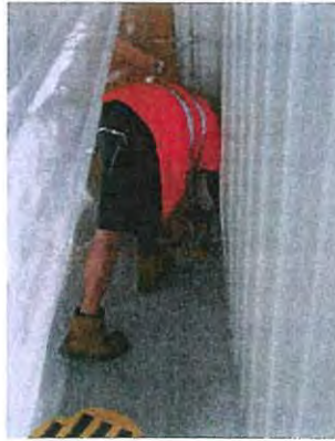
Fixing base of liner inside container
